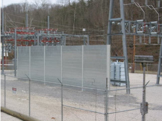
Engineered sound control wall installed
