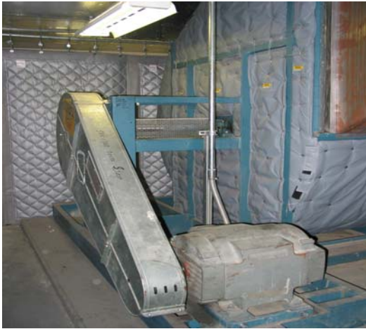
Blower casing shown with Unger's removable sound blanket
