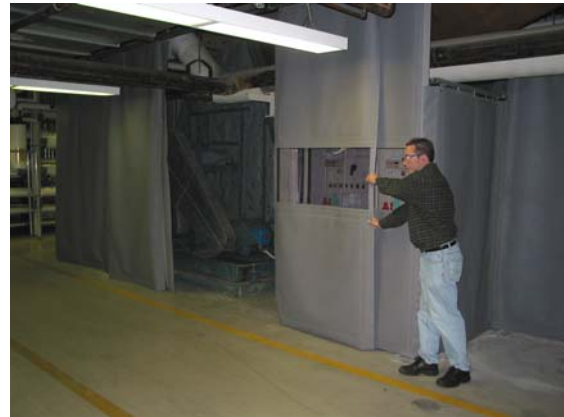
Fan shown with sliding access sound curtain
