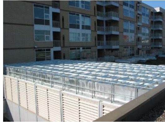
Outdoor Condenser Fan Noise Remediation
